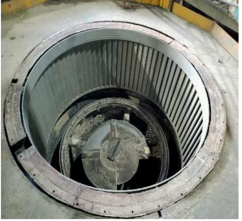
Newly Modified separator rotor installed.
