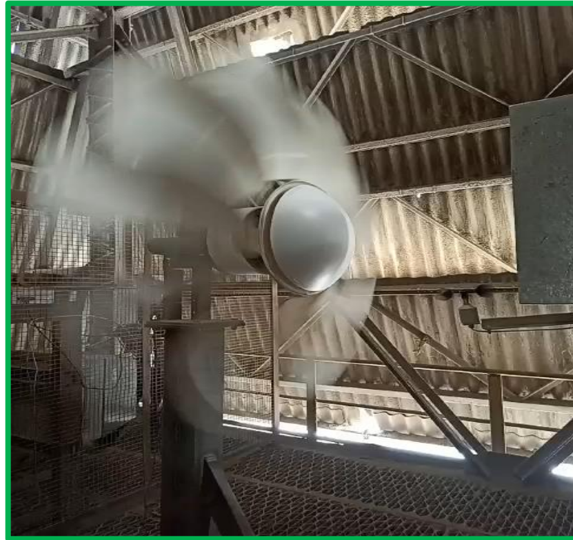
During Installation - UE 22 9 blade spherodynamic 3 KW Wind turbine
