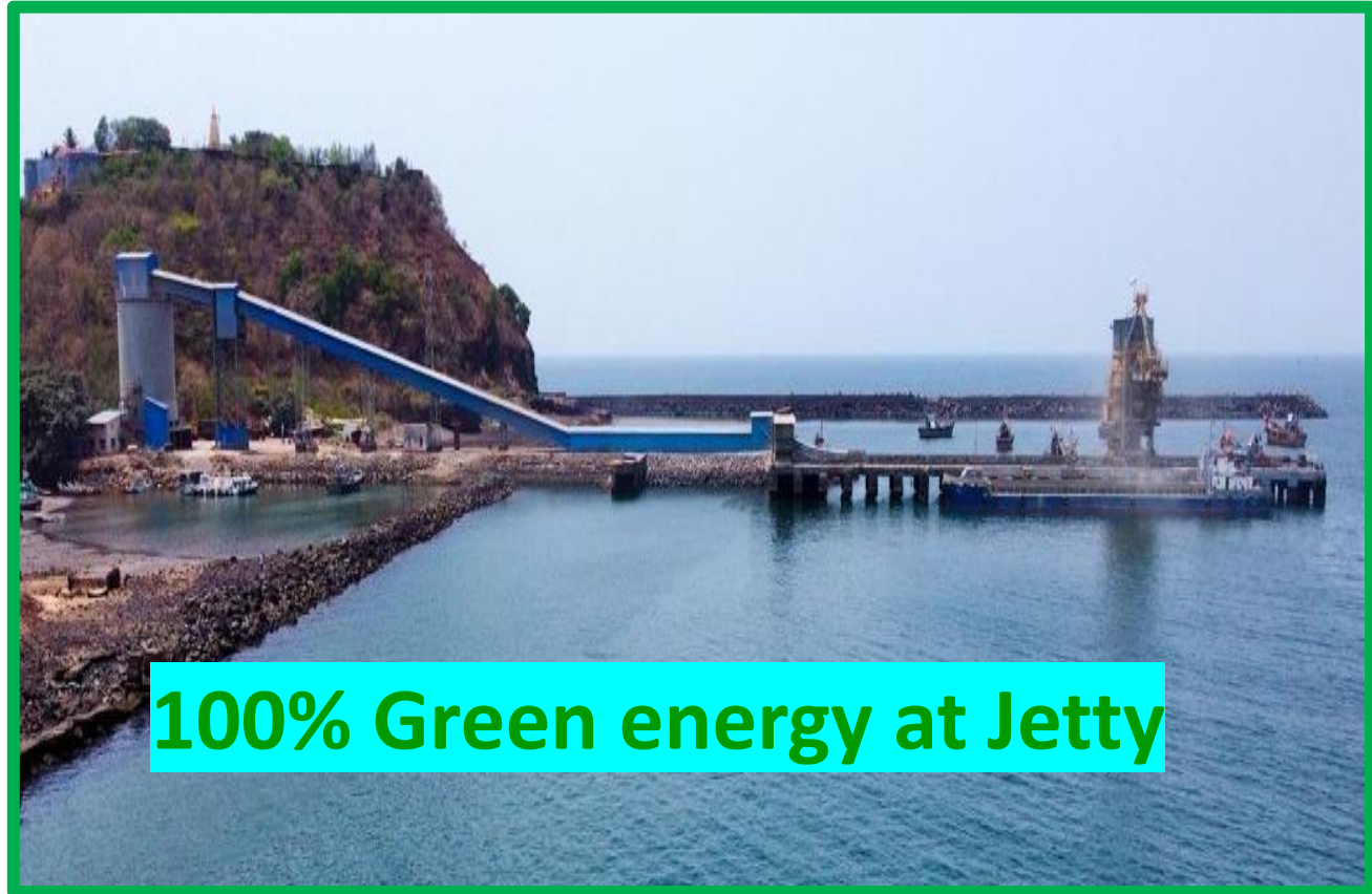
Entire Jetty is running on MSEDCL green power
